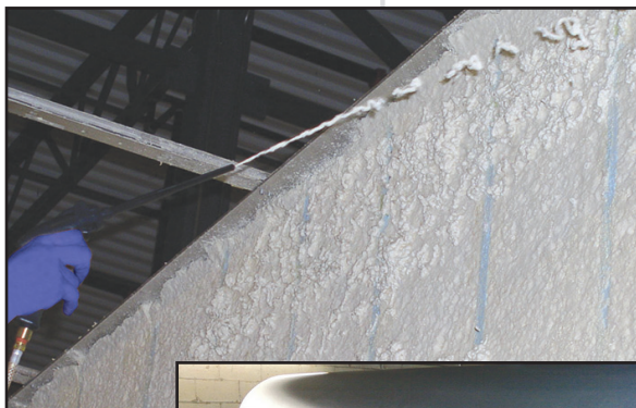
Side wall application
